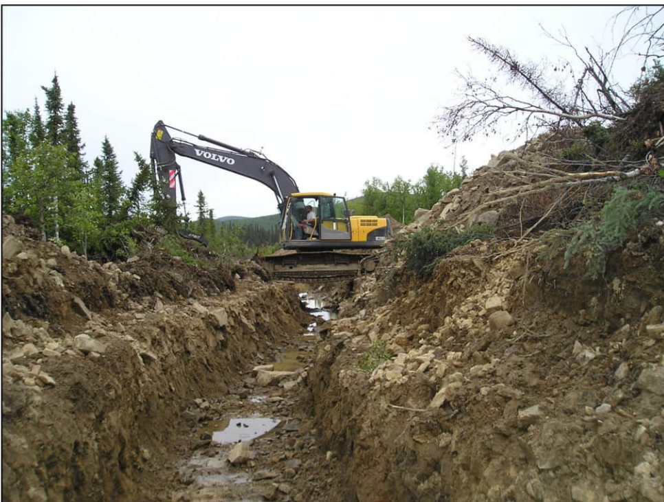
Photo 1. Excavator Trenching at Green Gulch
